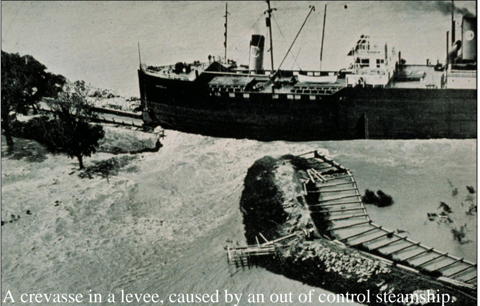
A crevasse in a levee, caused by an out of control steamship.
